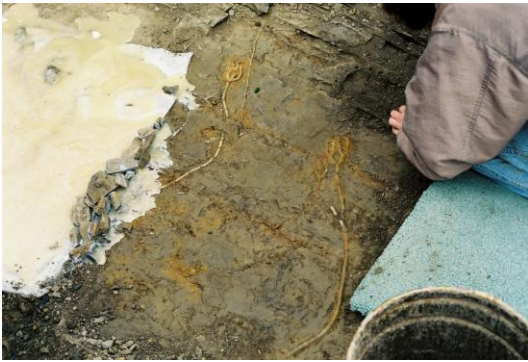
Epoxy glued area next to next slab.
